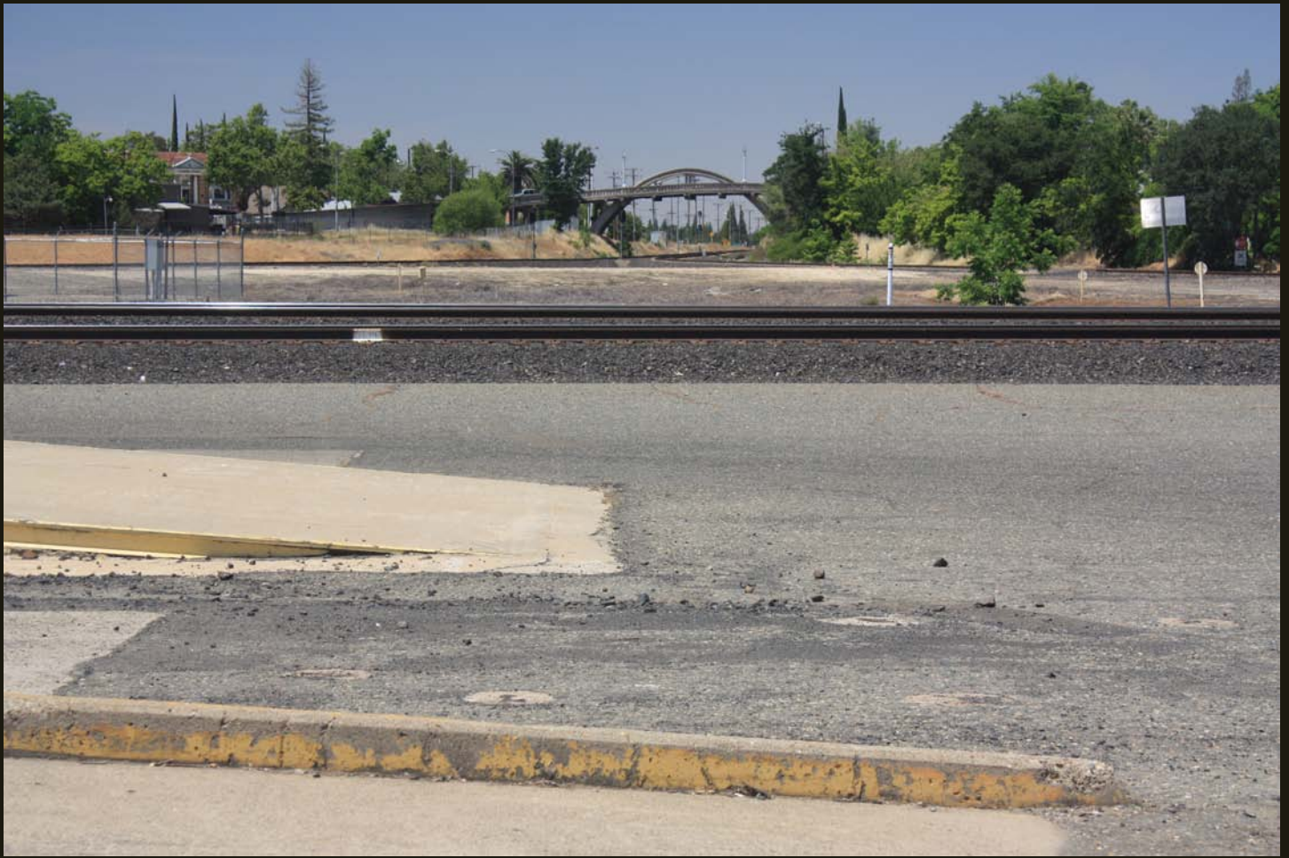
Northwestward view of the CP (1869) mainline in the foreground and the C&O (1872) wye in the distance. This is presumably the location of the crossing of the CC (1861) and the track beyond the tip of the wye (beneath the overpass in the distance) is on the alignment of the 5-foot-gauge CC. There is no evidence of the CC on the ground and I found no evidence of any major re-alignments; a 1908 topo map shows the wye in the same location as today.
