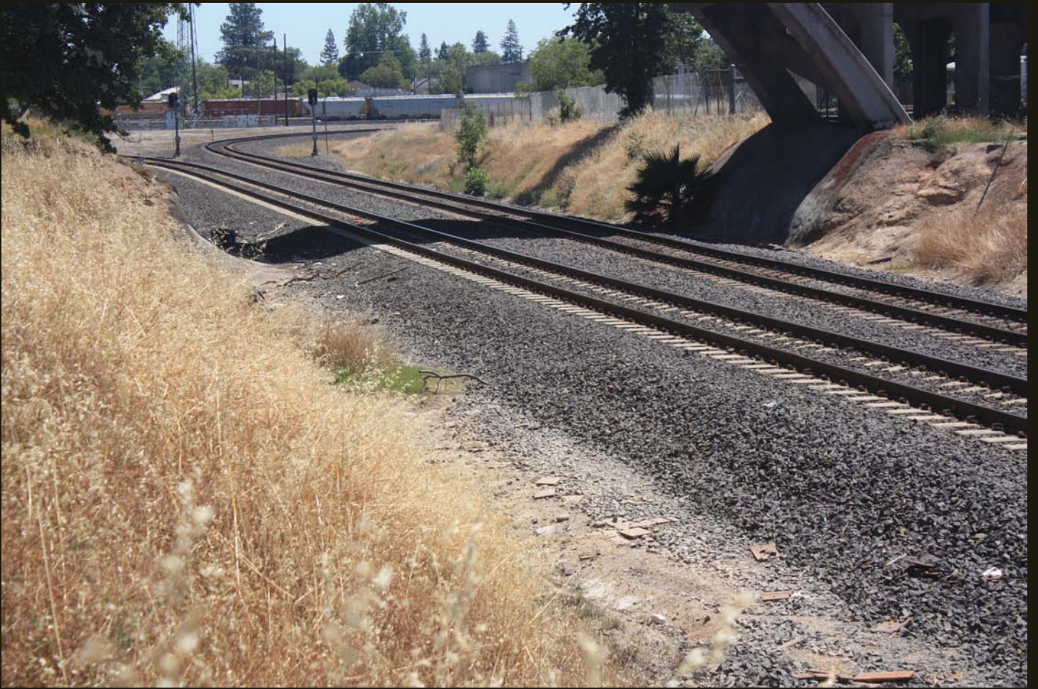
Another southward view of the C&O (1872) wye, the tip of which is two parallel tracks for a short distance.
