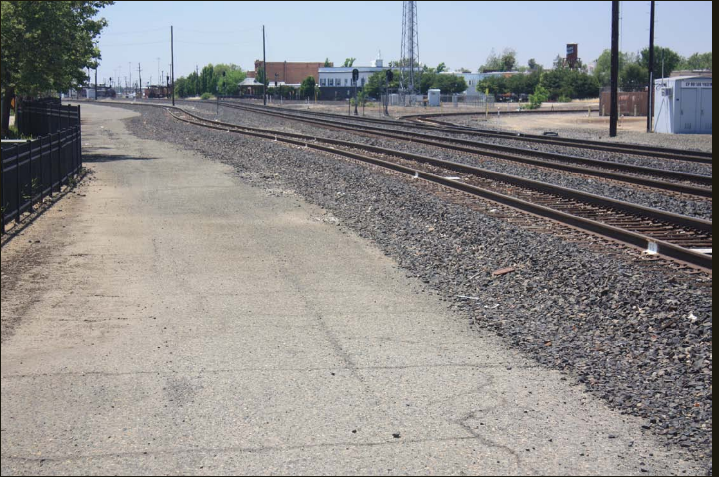
Westward view of the CP (1869) mainline in the foreground and the C&O (1872) wye veering off to the right (north).
