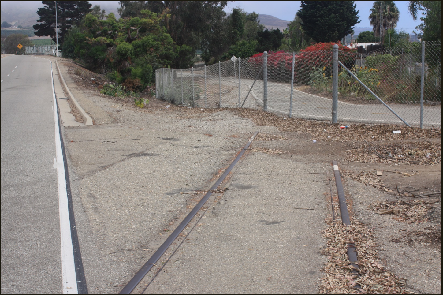
Northward view of the V&OV (1898) at far end of the track in the first photo. Beyond the fence the Ventura River Trail follows the railroad grade; the trail to the right of the nearest curve is on a new alignment to allow safe access for bicycles.
