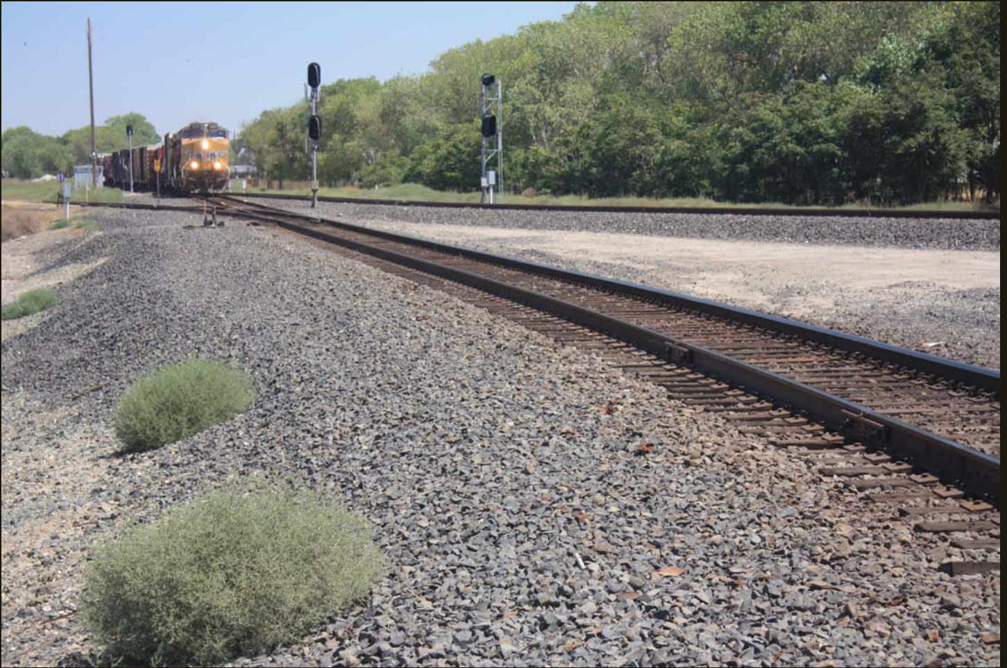
Westward view of the western tip of the SP wye. The front of the train is on the switch for the wye, which joins the two curved tracks of the wye, both bolted. The track to the left, with a switch in front of the train, is a spur to a junkyard (AMG Resources on the satellite image).
