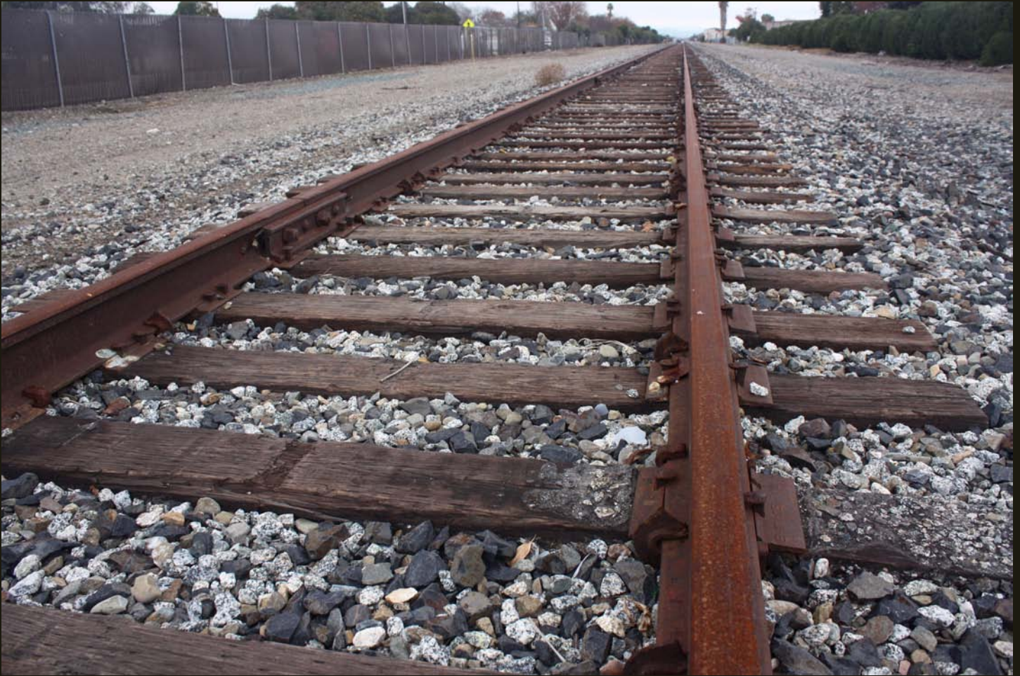
Northwestward view of the SP&T (1878) a half mile northwest of its junction with the WP (1869). The track is very rusty and I could find no documentation that the line was used in recent years.
