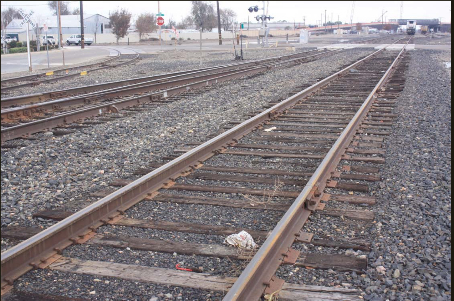
Northeastward view at the wye for the SP West Side Line (1891). The track in the foreground is the siding for the wye, the track to its left is the WP (1869) main line with a switch to its siding (with caboose and box cars out of the sight to the left), and the curved track to the left is the spur that heads 3 miles north from this location. The two sidings in the right distance are for the east branch of the SP West Side Line (1891) wye, which today is the busy interchange between the California Northern Railroad, which operates on the SP West Side Line (1891) line, and UP, which operates on the WP (1869) line.
