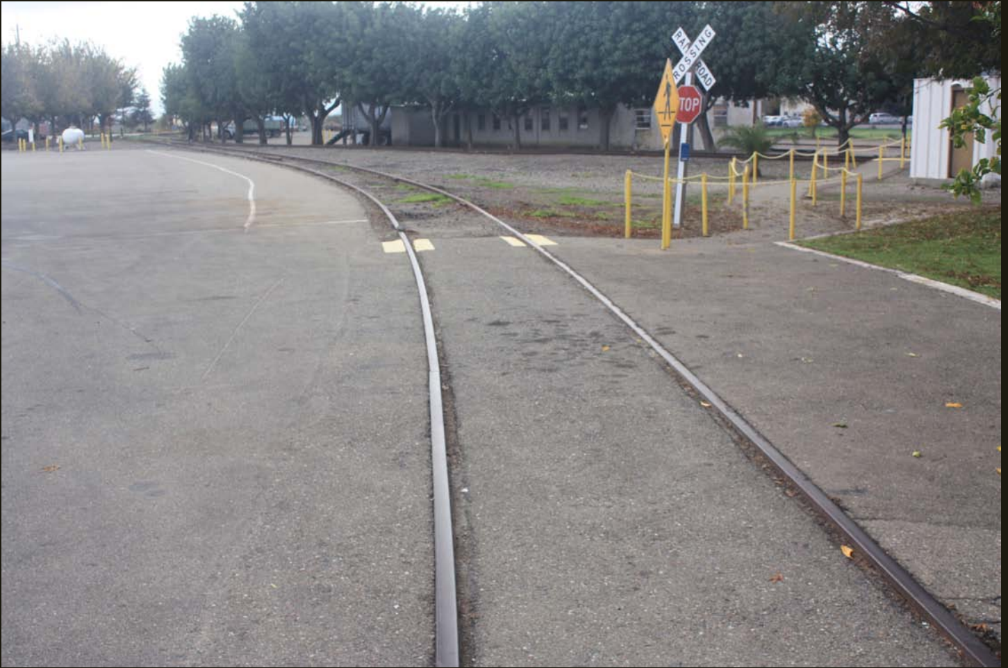
Southwestward view of the east branch of the Carbona wye, which was built at the time or soon after the A&SJ (1896) was re-aligned to accommodate the WP (1909).
