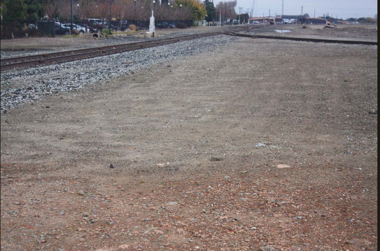
Northeast view at same location as previous. The bolted WP (1869) line is on the left and the parked cars farther left are for the City of Tracy Transit Center. The switch and curved track to the right is a 1.5-mile-long spur.
