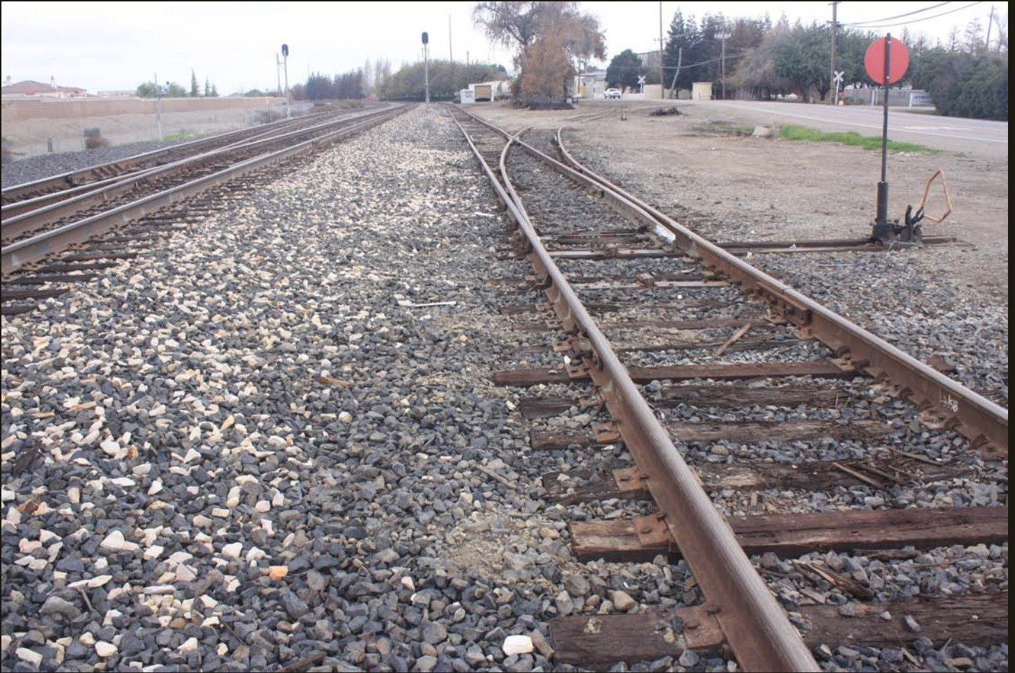
The west branch of the Carbona wye is in the right foreground, and the WP (1909) main line and siding converge to one track on the left.
