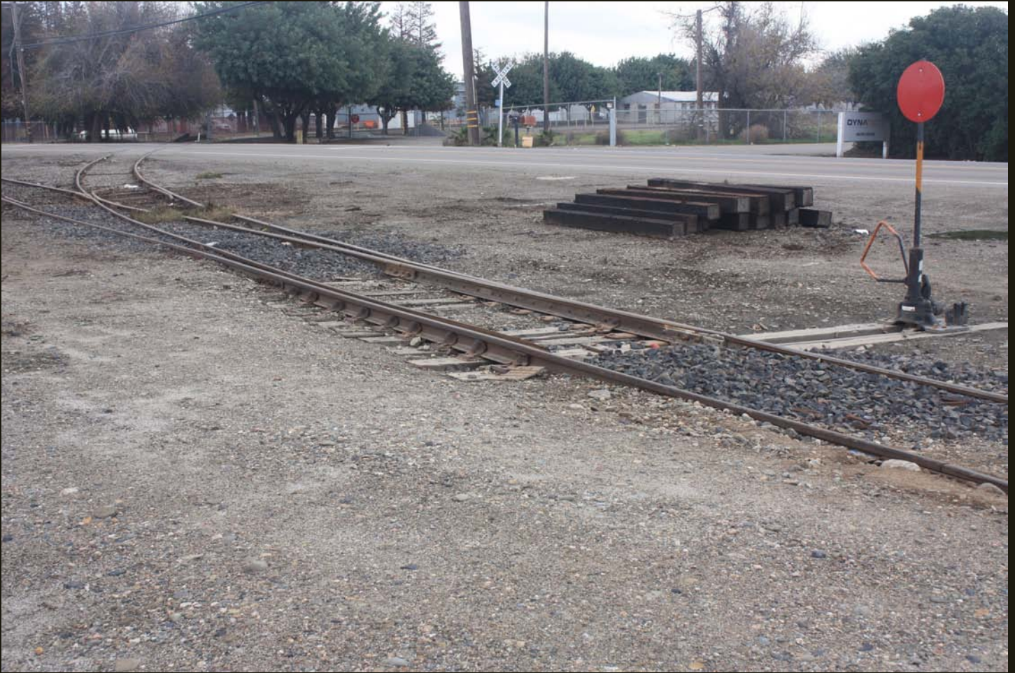
Southeast view of the west branch of the Carbona wye and its junction with the siding.
