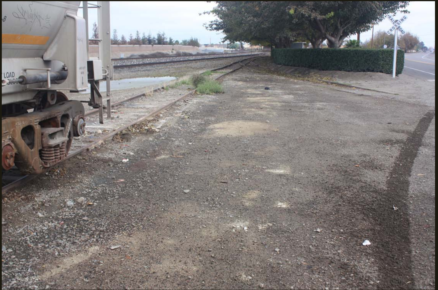
Northeastward view of the east branch of the Carbona wye (curved track on right) where it merges with a siding of the WP (1909), which is the higher track in the distance. The curved main line in the distance marks the transition of the WP (1909) alignment from the northeast-southwest alignment of the A&SJ to the east-west alignment of WP (1909) new grading in the foreground.
