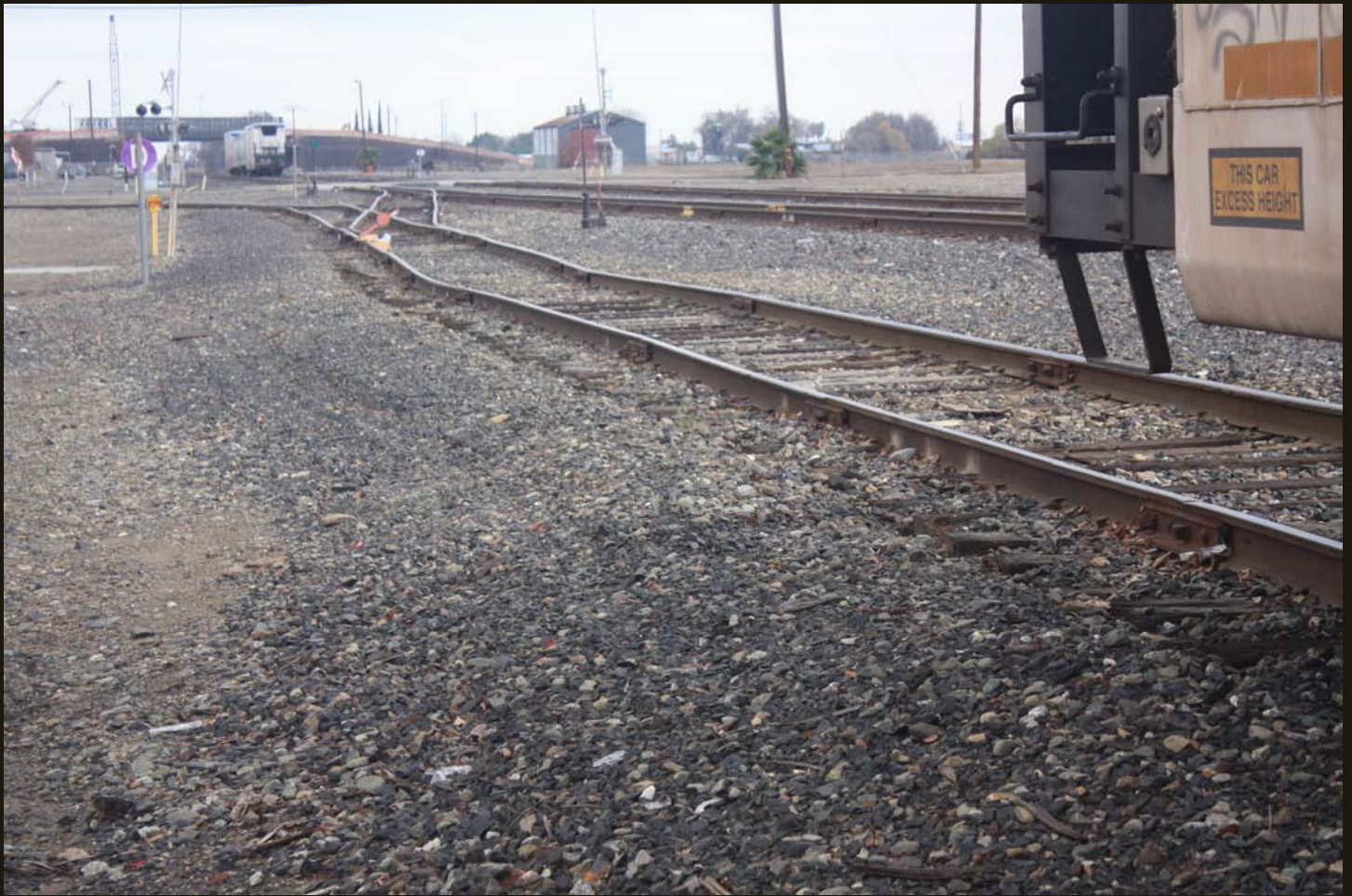
Eastward view at the wye for the West Side Line, the nearby box car in the upper right is the easternmost box car on the WP (1869) siding (previous photos). The siding branches to the right onto the WP (1869) main line and to the left onto a spur that heads 3 miles due north from this location.
