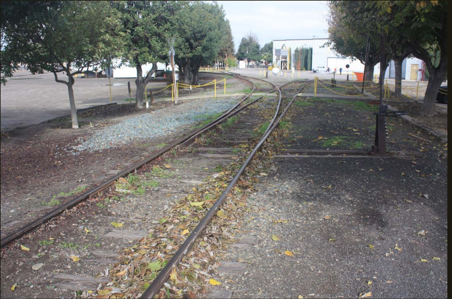
Northward view of the Carbona wye, the switch in the previous photo is now in the distance, the nearer switch is a spur to the warehouse in the distance.
