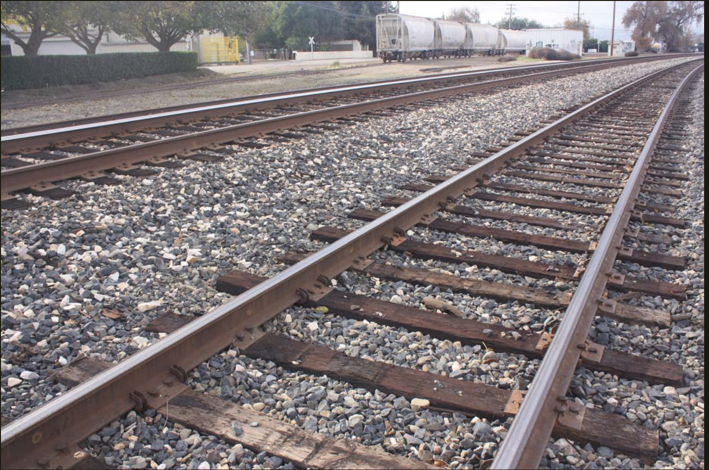
Southwestward view a few step from the previous location. The WP (1909) main line is in the foreground, turning from its southwestward A&SJ alignment to its westward new alignment. The next track to the left is a siding, and the siding with cars stored is for the Carbona wye.
