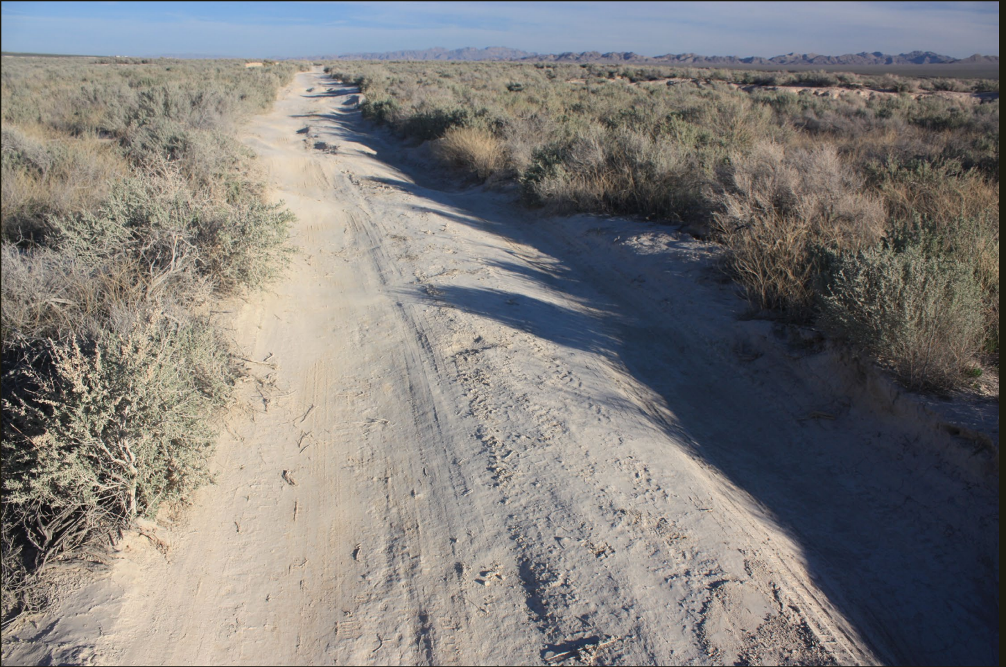
Northwestward view of the LV&T (1907) near Corn Creek, same location as previous. The LV&T grade has been used as automobiles for nearly a century but is not significantly re-graded. The grade climbs for another 25 miles to the northwest before it crosses the drainage divide between the Colorado River (including Las Vegas and this location) and the Great Basin.
