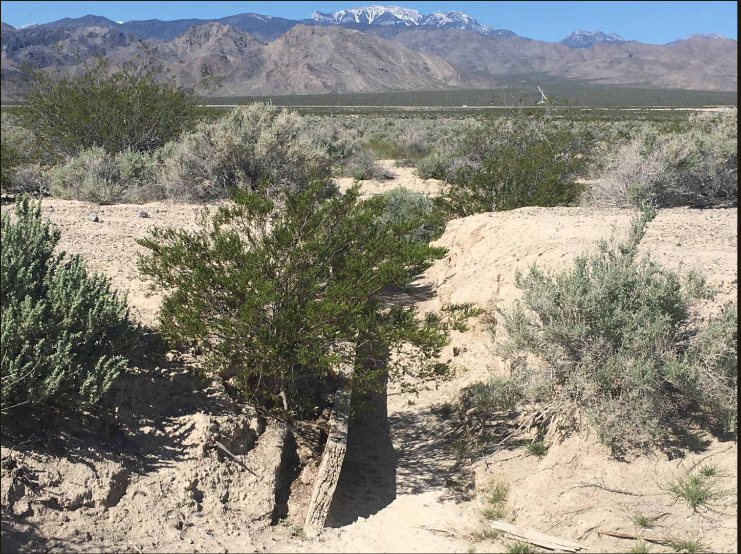
Southwestward view of the LV&T (1907) near Corn Creek, 1/4 mile northwest of the previous location. The slab of wood in the foreground was once part of a culvert to allow drainage beneath the railroad fill grade; I've seen identical culverts on the nearby Tonopah and Tidewater (1907), which was built at the same time as the LV&T (1907).
