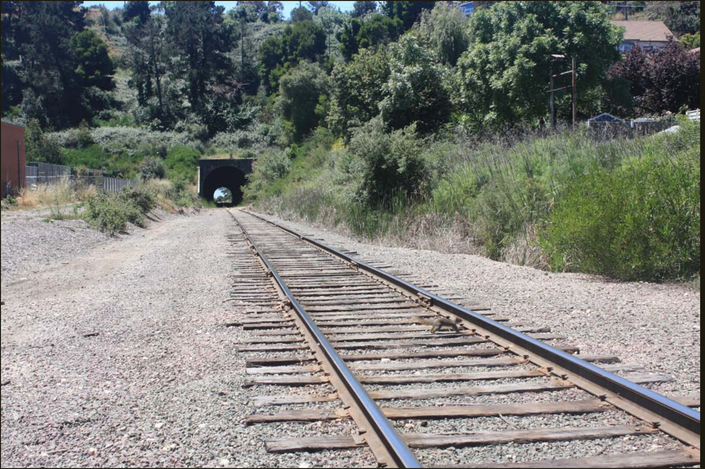
Southwestward view of the SF&SJV (1900), same location as previous. To access the location of the ferry landing at what became Ferry Point on the larger Point Richmond, the AT&SF had to build this tunnel through the Potrero San Pablo Ridge. Commercial use of the ferry ended in 1975 and the ferry facilities burned in 1984. The track is usable only to the tunnel and the end-of-track at the former ferry pier is a mile down the line.
