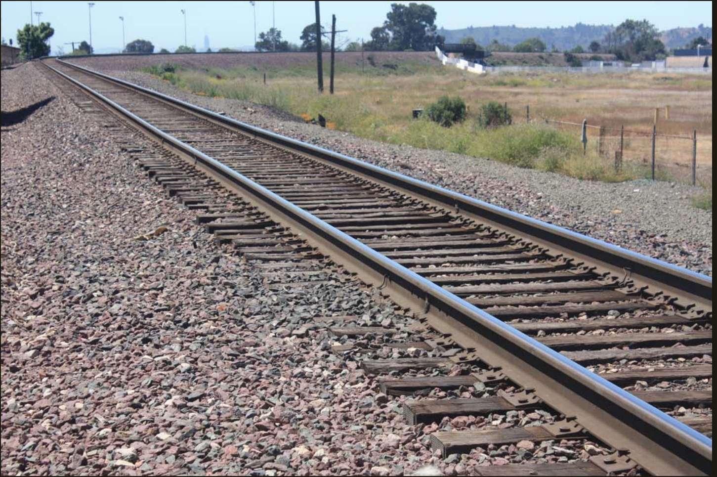
Southwestward view of the SF&SJV (1900), 300 feet south of previous location. Note the rising fill grade and bridge over the SP&T (1878) (just right of center) grade crossing as the SF&SJV alignment turns southwestward toward Richmond.
