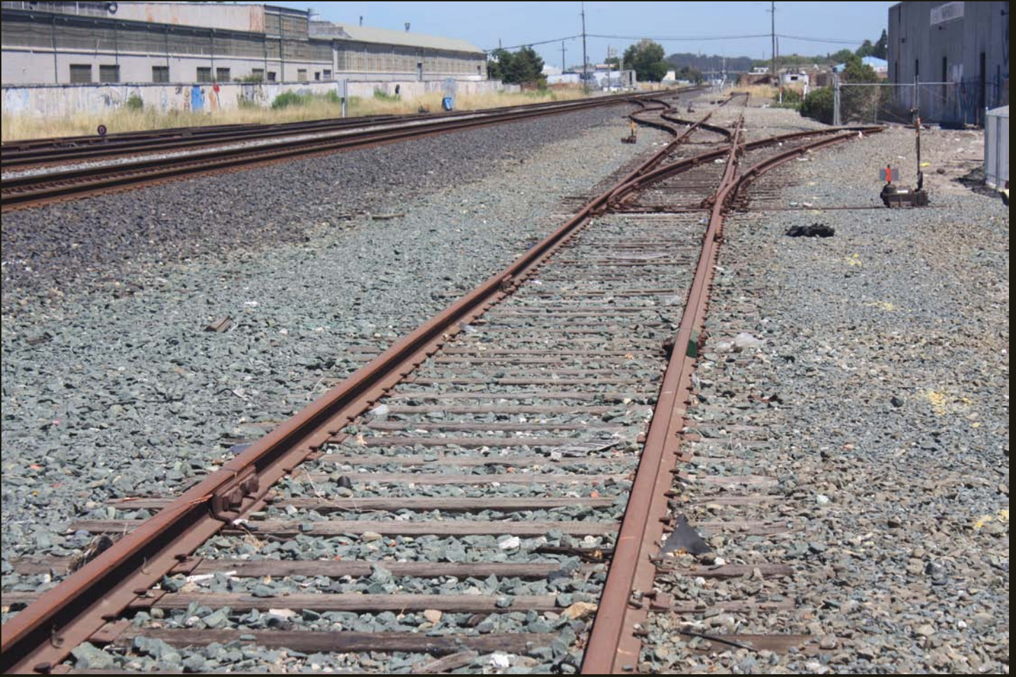
Northward view of the SP&T (1878) and sidings, a quarter mile north of its crossing of the SF&SJV (1900). Note the weird Ben and disconnection in the middle of the crossover trap; this indicates the former presence of another other track in the middle.
