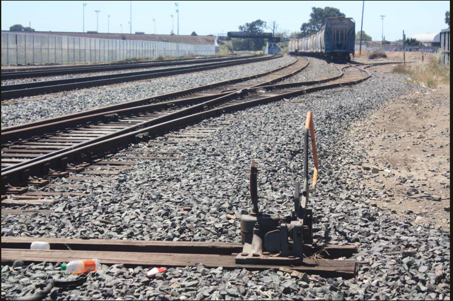
Southward view of the SP&T (1878) and its crossing of the SF&SJV (1900). The branch to the right (west) connects the SP&T/SP (now UP) to petroleum and port facilities 3 miles to the west, just north of Richmond at San Pablo Point. The overpass is the SF&SJV/AT&SF line to Richmond, which we will explore below.
