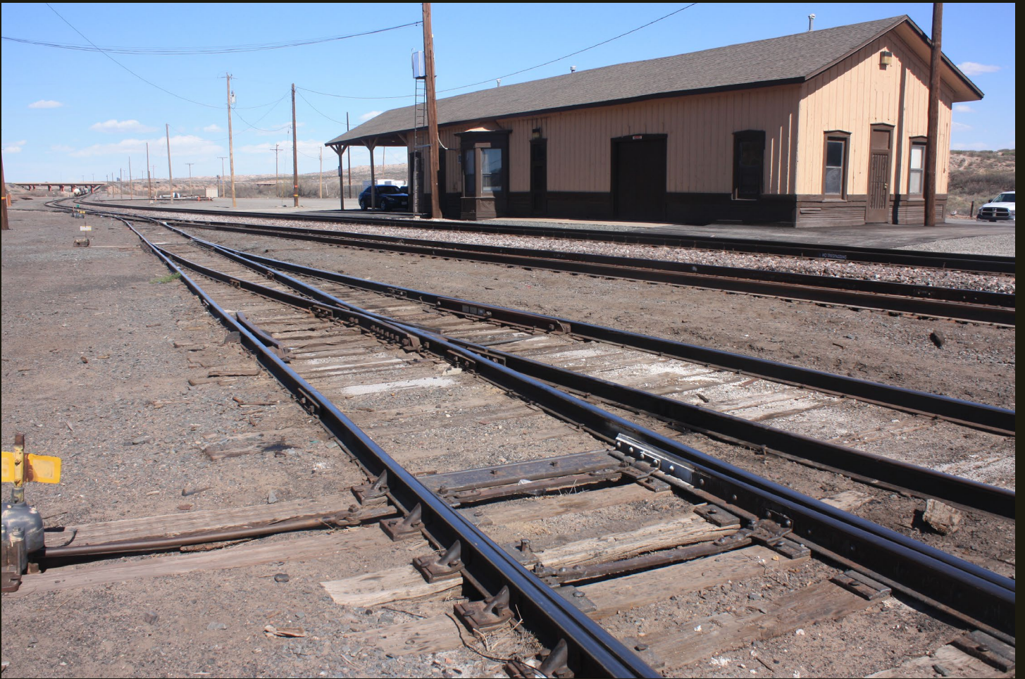
This building in the Rincon yard does not look like an original station and appears to be a modern operations facility.
