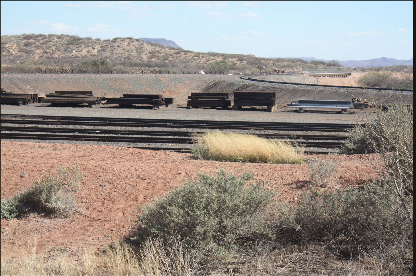
Southeast view of the Rincon wye. The sidings and route in the foreground is the AT&SF's RGM&P (1881) line to Deming and the branch forming the wye is the AT&SF's RGM&P (1881) line to El Paso.
