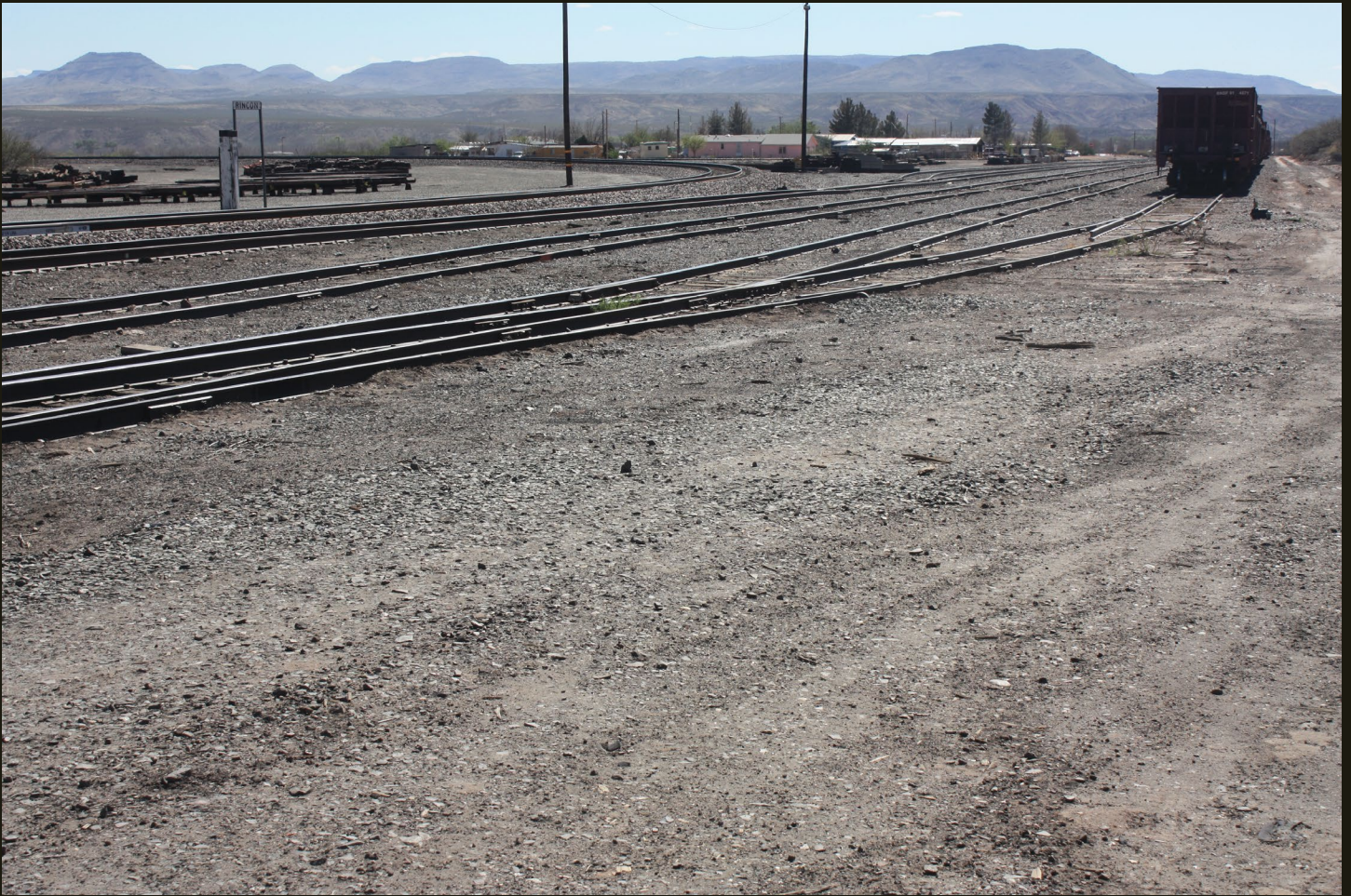
The yard at Rincon. The sidings and route to the right (southwest) is the AT&SF's RGM&P (1881) line to Deming and the branch to the left (southeast) is the RGM&P (1881) line to El Paso.
