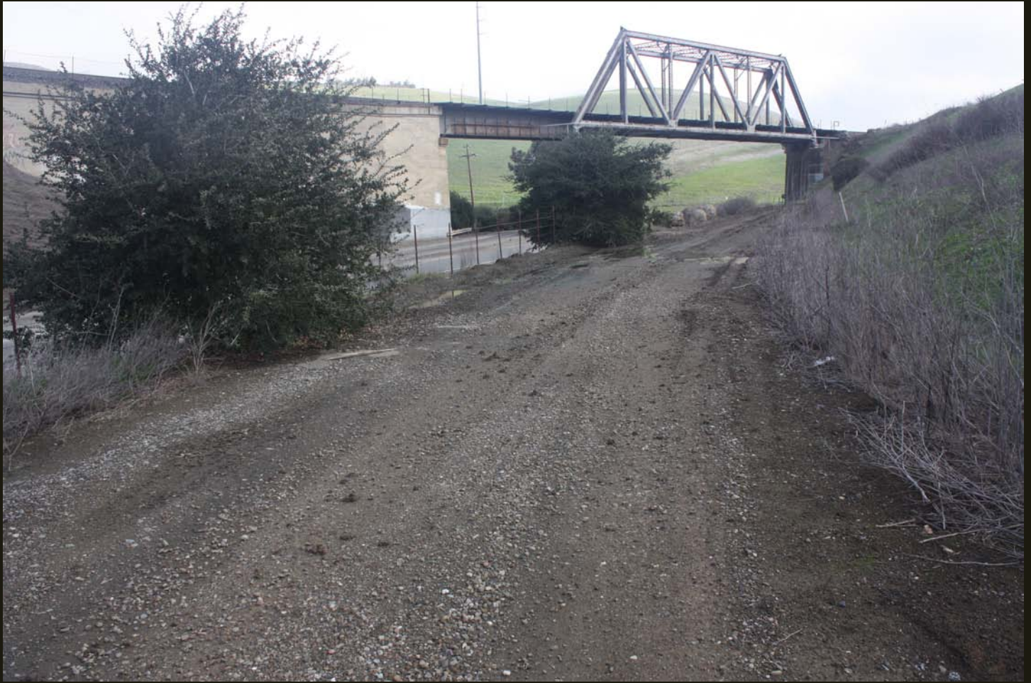
Eastward view one-half mile east of Altamont Pass. The abandoned WP (1869) grade again passes under the WP (1909) tracks to follow a steeper grade down to the valley.
