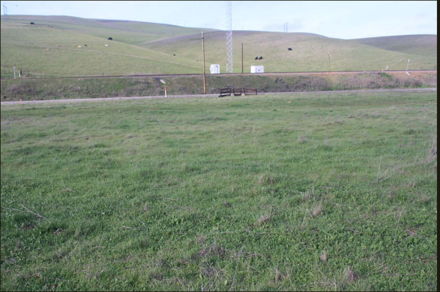
Northwestward view 2 miles west of Altamont Pass. The abandoned WP (1869) grade is lower and closer with a small culvert; the WP (1909) tracks are on a higher fill grade.
