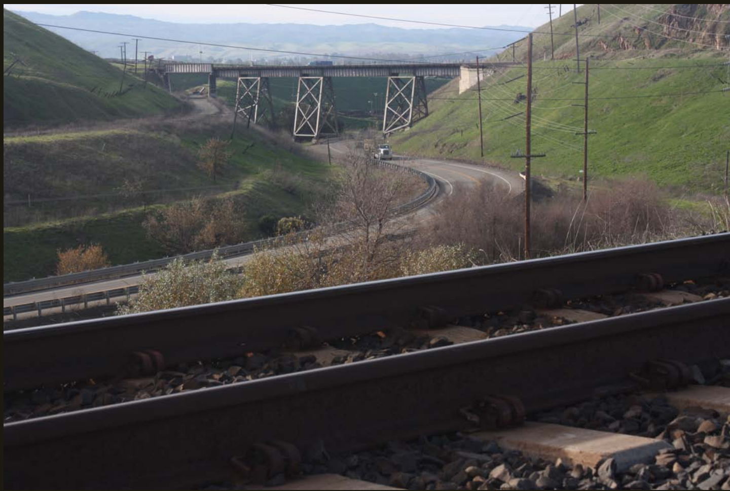
Westward view of the same WP (1909) bridge as the previous photo. The abandoned WP (1869) grade is steeper and so passes under the bridge on its approach to Altamont Pass.
