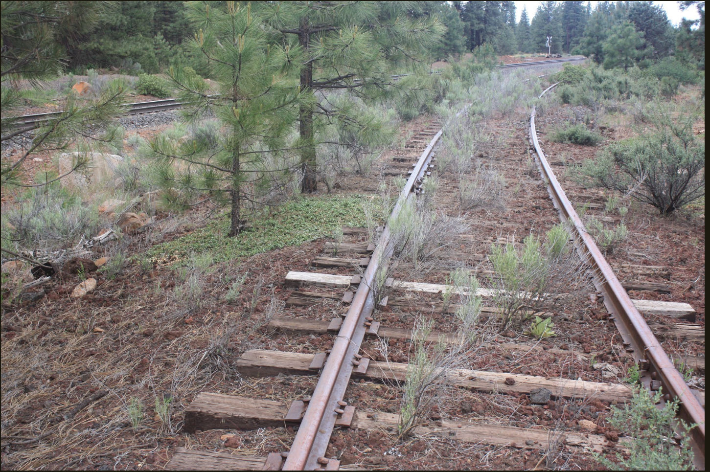
Southeastward view of the loop line, 200 feet northwest of the previous location.
