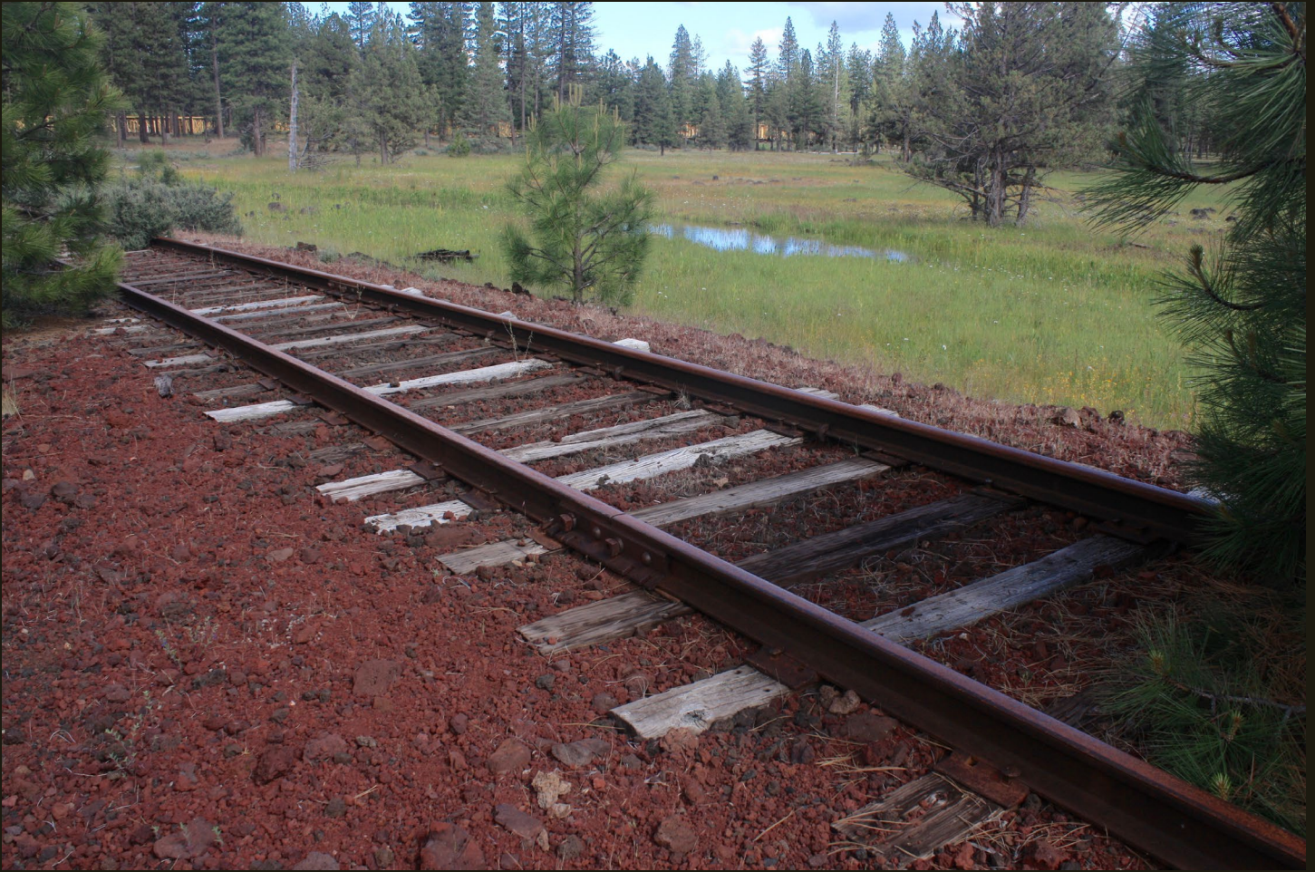
Eastward view of the loop track, same location as previous. Note the red ballast rock, which is volcanic cinder, a common rock type in northeastern California. Note also, through the distant pines, the same stored cars on sidings of the Inside Gateway (now BNSF) mainline.
