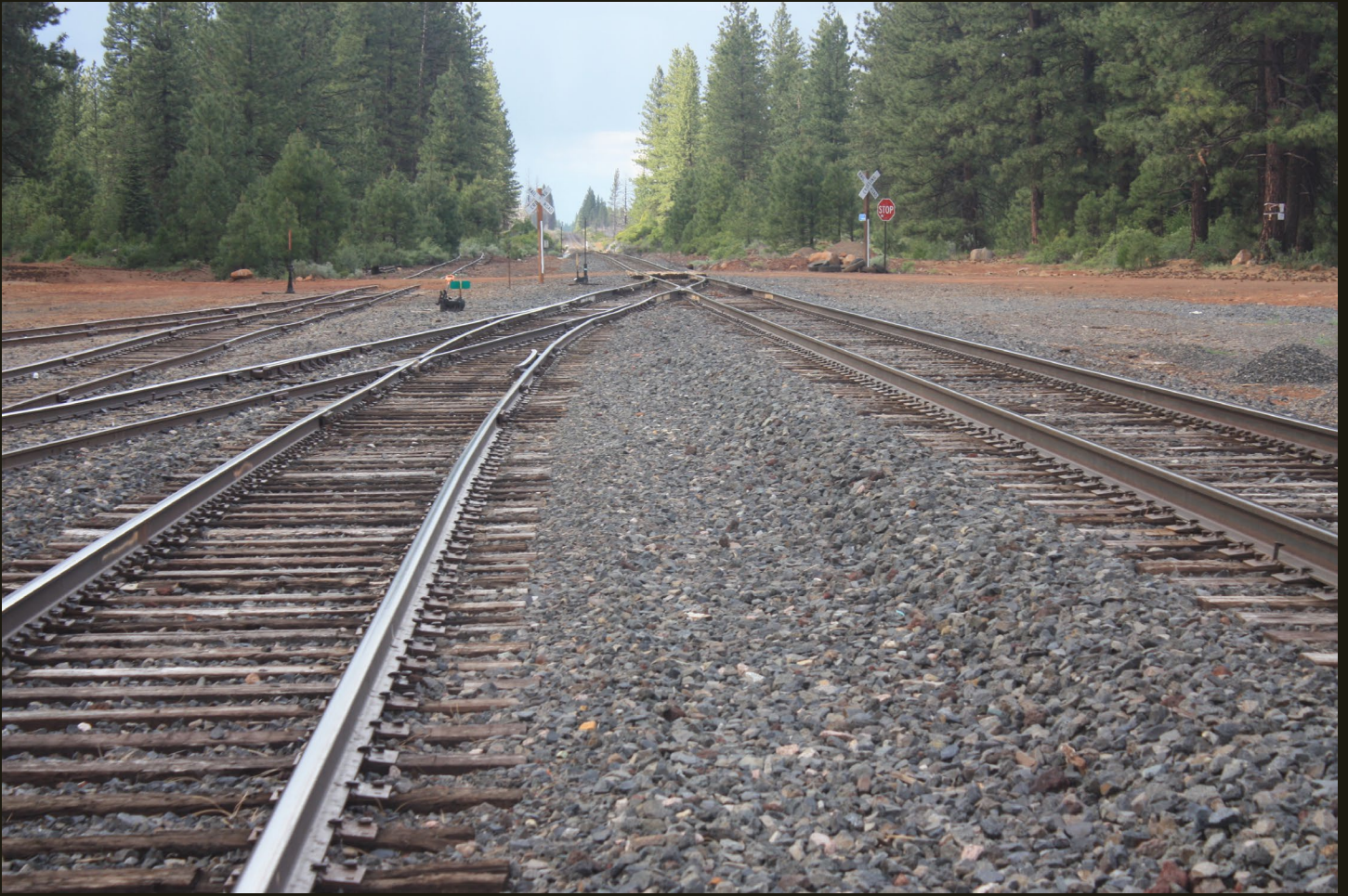
Northward view of the GN Inside Gateway (1931) a few steps north of the previous location; the shed is just out of sight to the left. From left (west) to right the tracks are: the loop line track (Hamburg Branch), including the south branch of the loop (far left) and its connection to the north branch of the loop line, which can be seen curving to the left in the distance and will be explored in the remainder of this geolink; the crossover track; the primary siding; and the Inside Gateway mainline.
