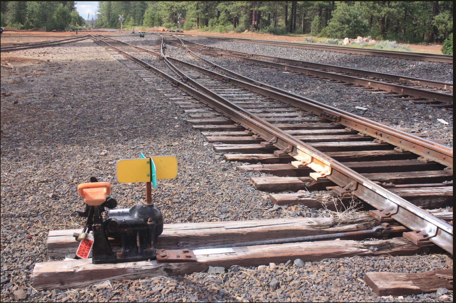
Northward view of the GN Inside Gateway (1931) a few steps west of the previous location. The closest line is the loop line and the switch is for the crossover to the loop line. The branch to the left is the southern part of the loop; the shed is just out of sight to the left.
